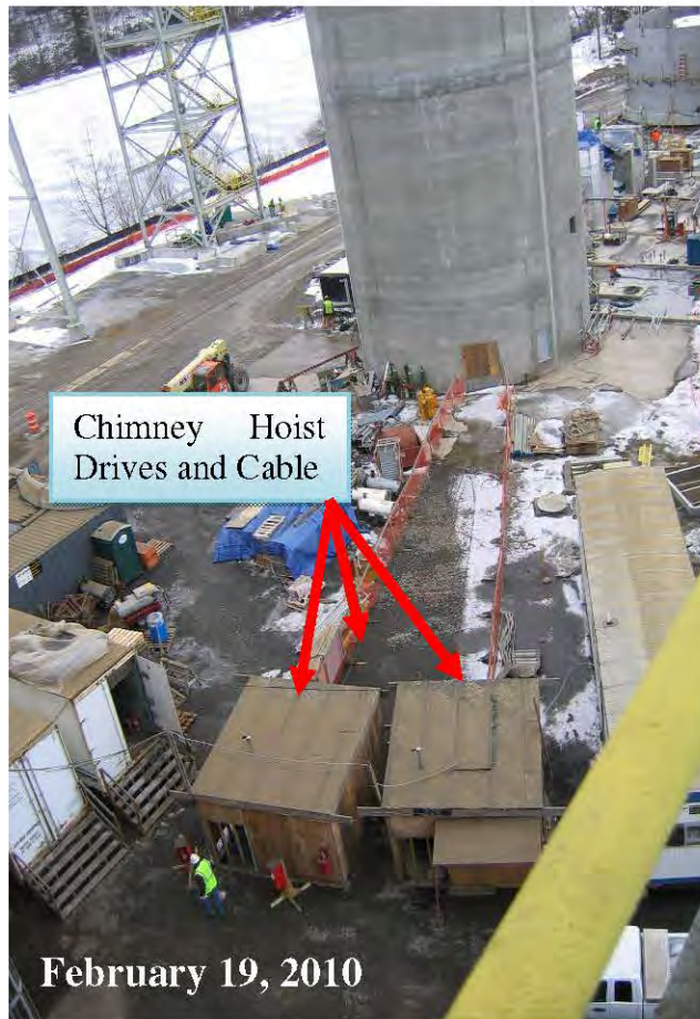
Figure 3 Chimney Hoist Drives and Cab (must be removed to install Booster Fan Foundation)
