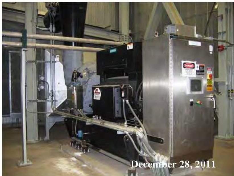
Figure A-6 Oxidation Air Compressor
