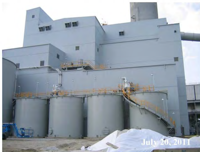
Figure A-4 South Side of FGD Building and Field Erected Tanks
