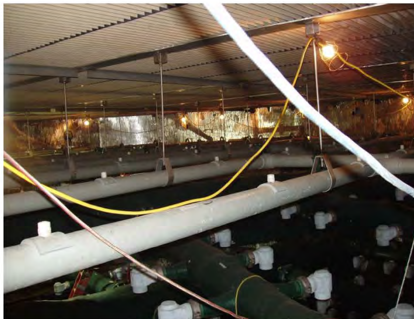
Figure A-6 View Inside the FGD absorber; slurry spray nozzles at bottom, demister spray piping in the center, and demister material installed at the top
