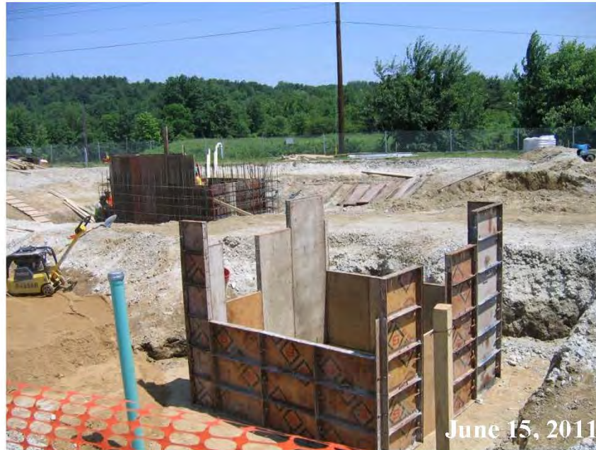
Figure A-1 SWWT System Foundations
