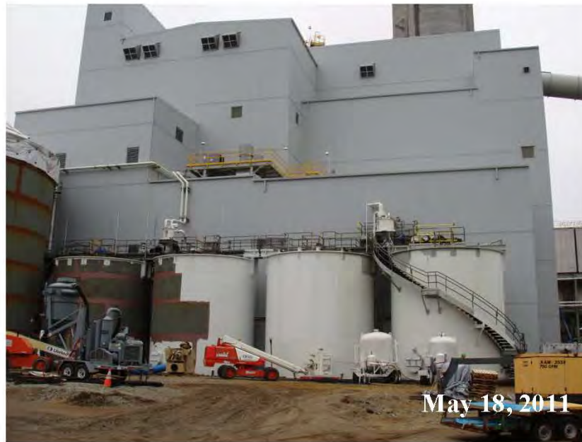
Figure A-1 FGD Building Looking North at Tanks being Coated
