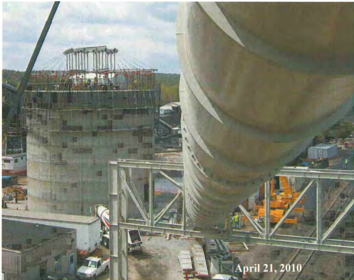
Figure 9 – Limestone Silo Erection and Limestone Conveyor L-3
