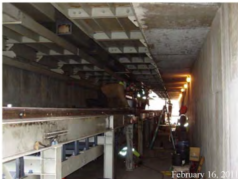
Figure A-10 Installation of Reclaim Shelf and Rotary Plow Track under Limestone Silos
