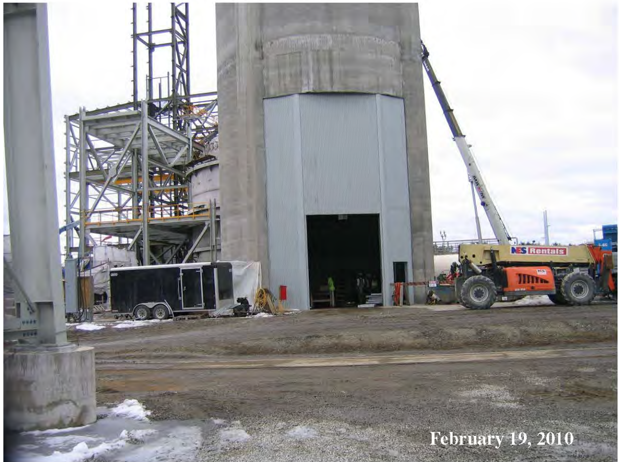
Figure 4 Chimney Enclosure Installation
