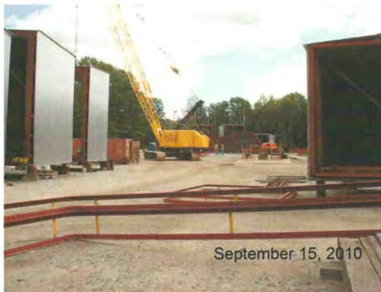
Figure 8 - Flue Gas Ductwork Ground Assembly
