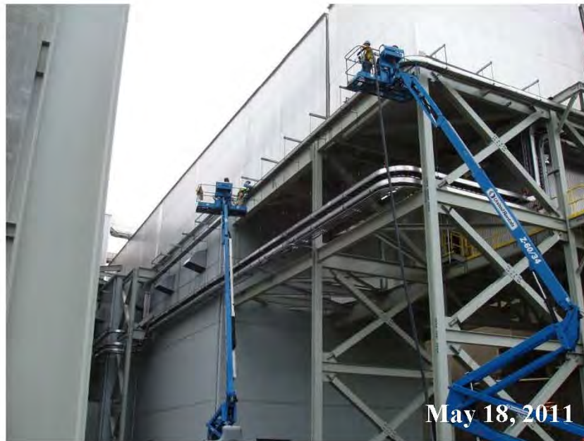
Figure A-3 Cable Pulling Near the Booster Fan Enclosure (looking northwest)
