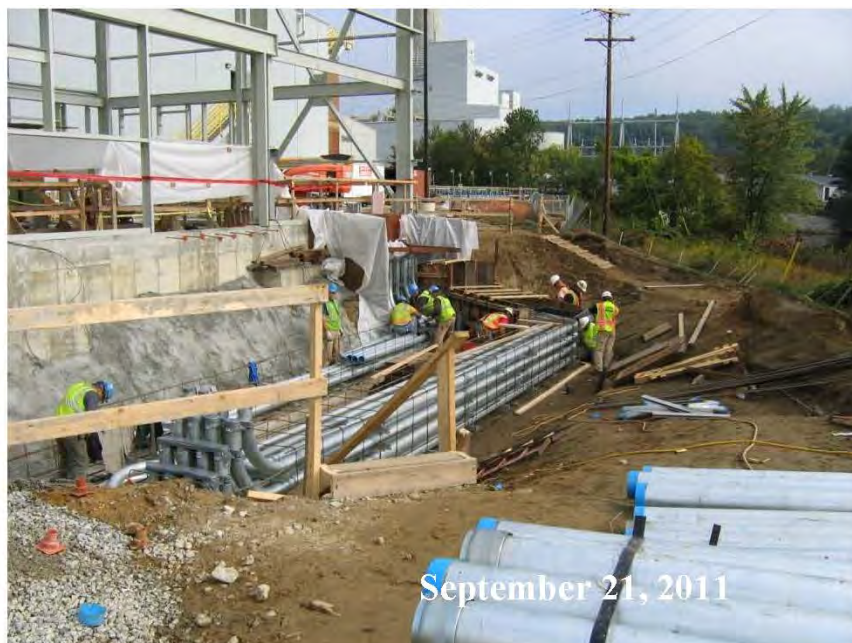
Figure A-2 SWWT Underground Electrical Conduit Installation
