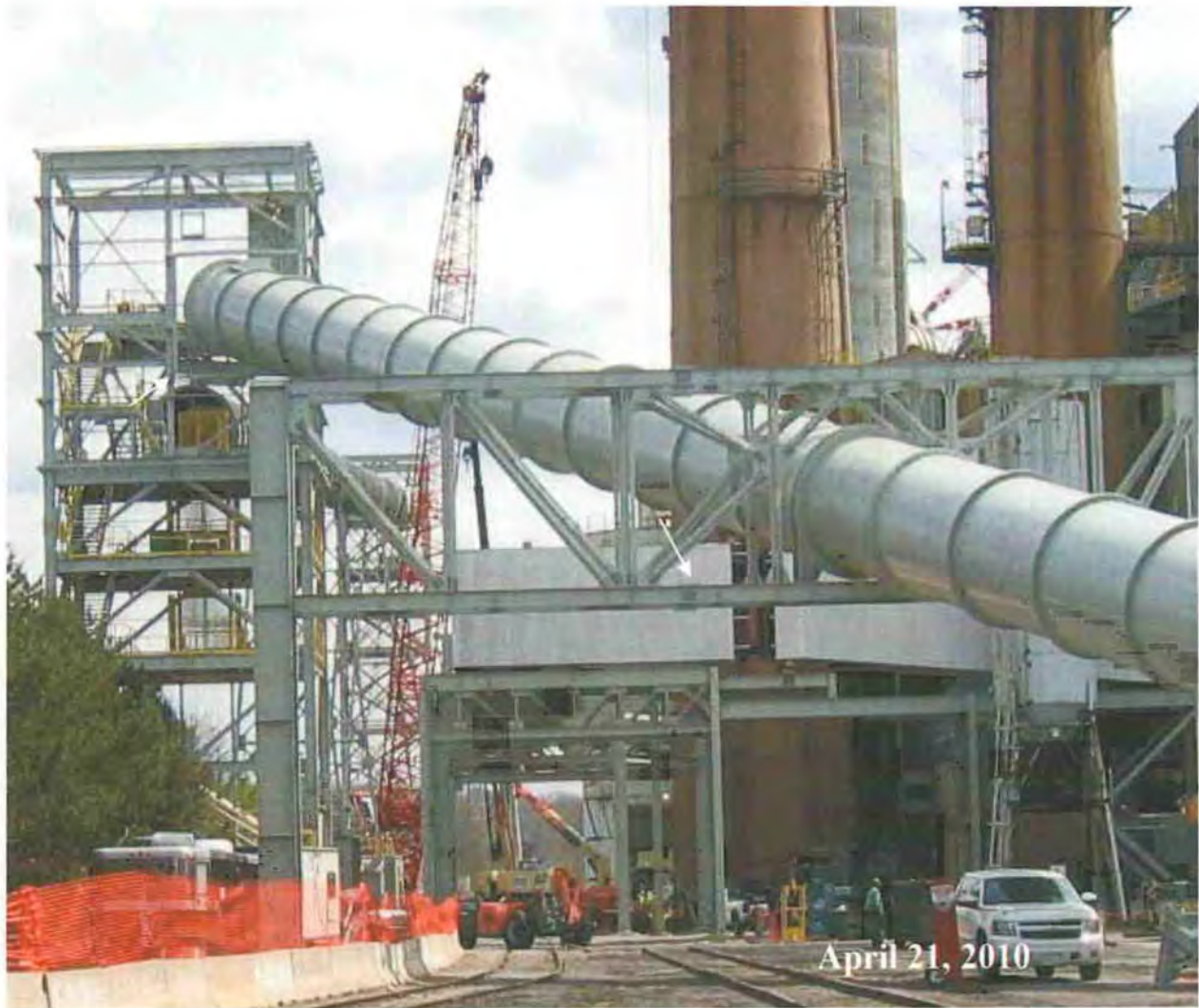
Figure 10 – Limestone Conveyor L-3 and Flue Gas Steel Ductwork
