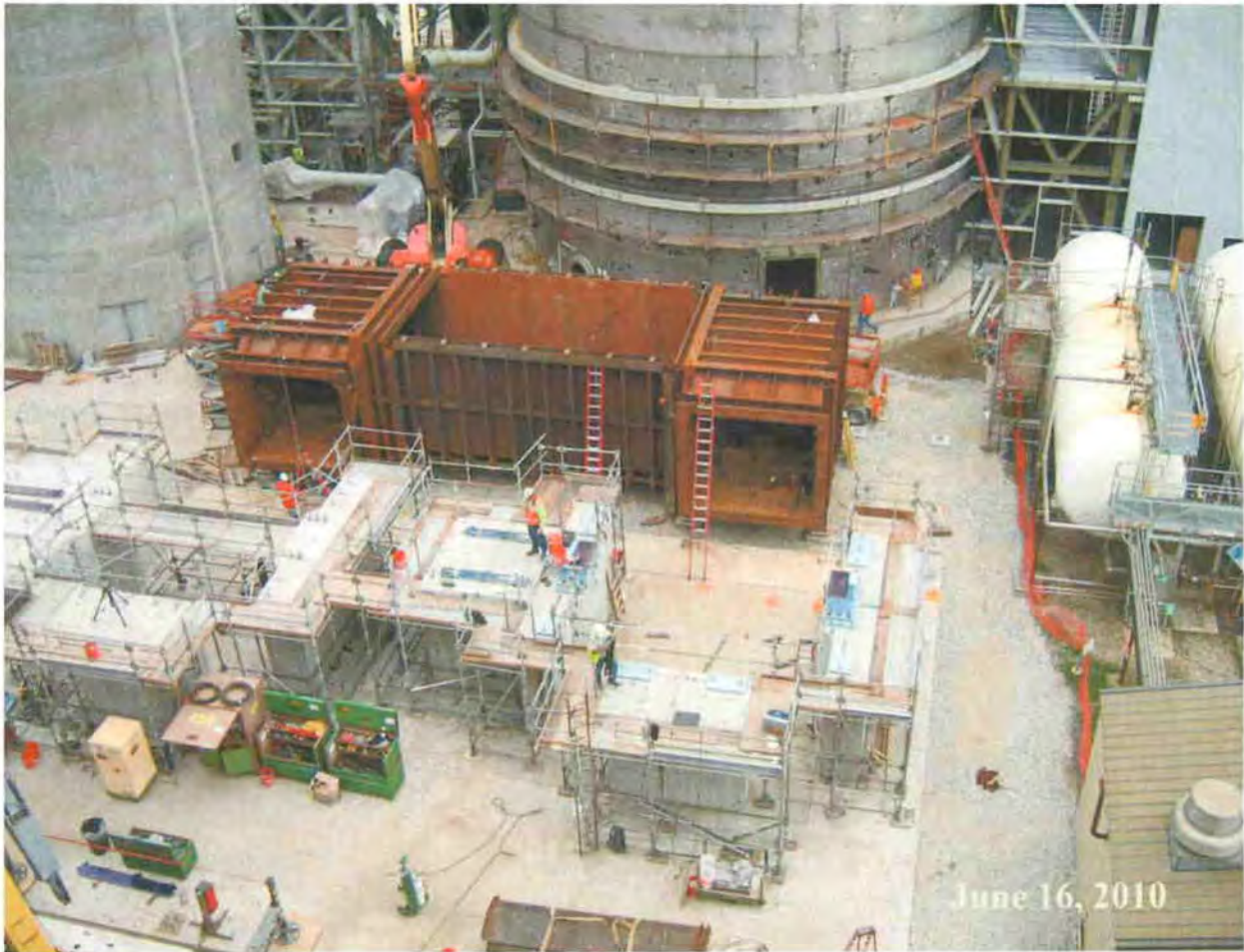
Figure 4 –Unit 2 Booster Fan Foundations and Ductwork
