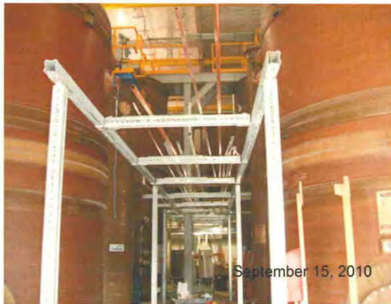
Figure 1 – Interconnecting Piping Installation in the WWR Electric Room
