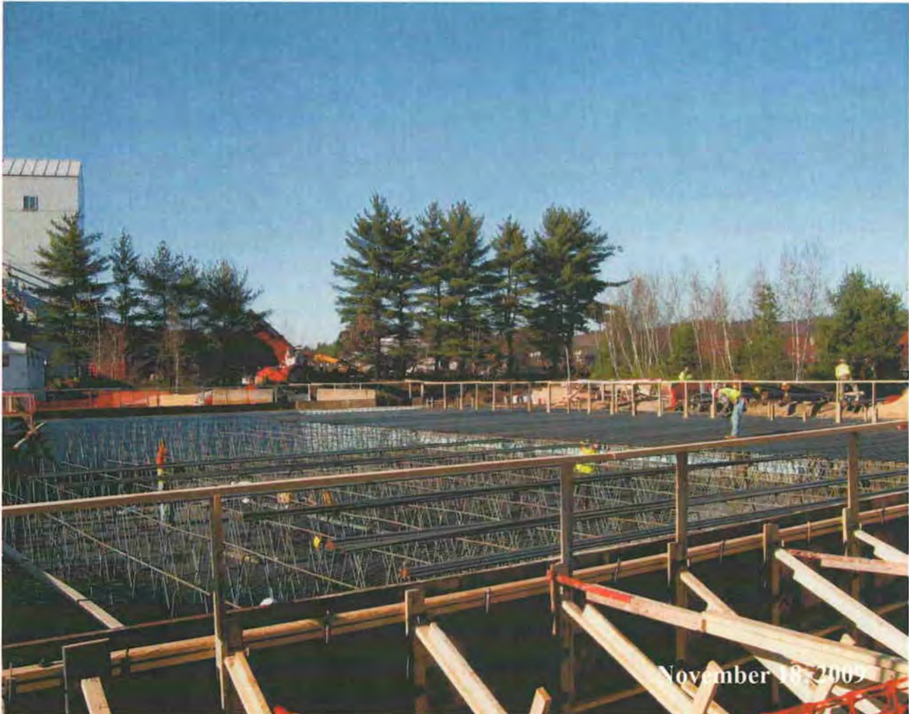
Figure 9. Foundation for Limestone Silos
