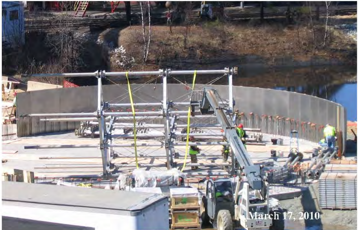
Figure 8 - Limestone Silo Erection
