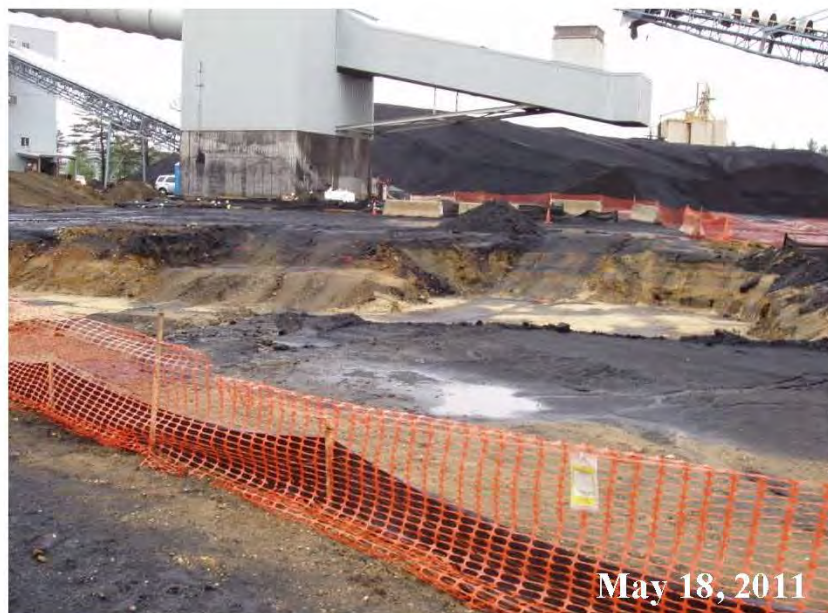
Figure A-7 LTDF Foundation Excavation
