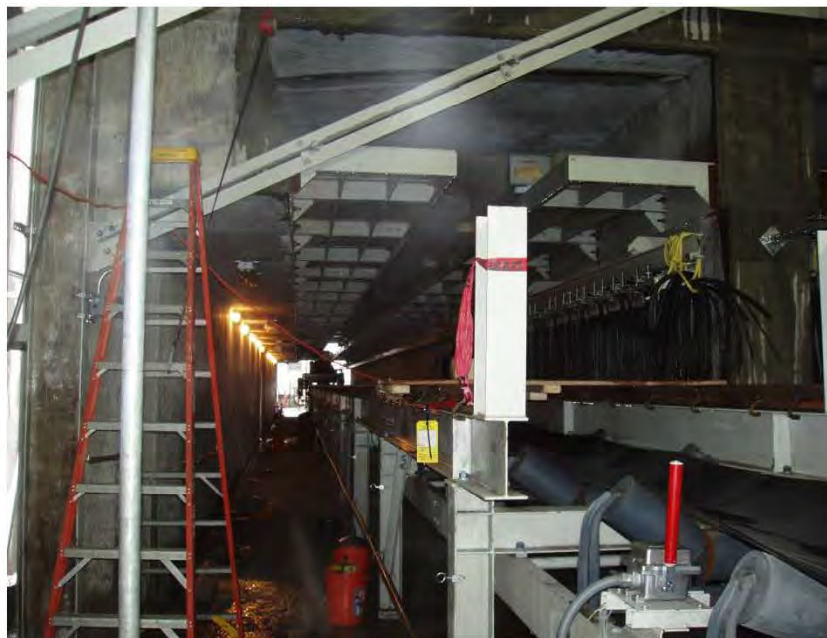
Figure A-10 Adjustment of reclaim shelf (rotary plow on track at far end) under limestone silos
