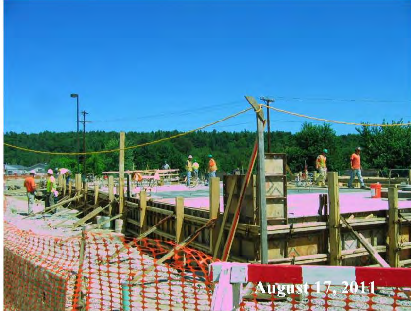
Figure A-1 SWWT Building Foundations
