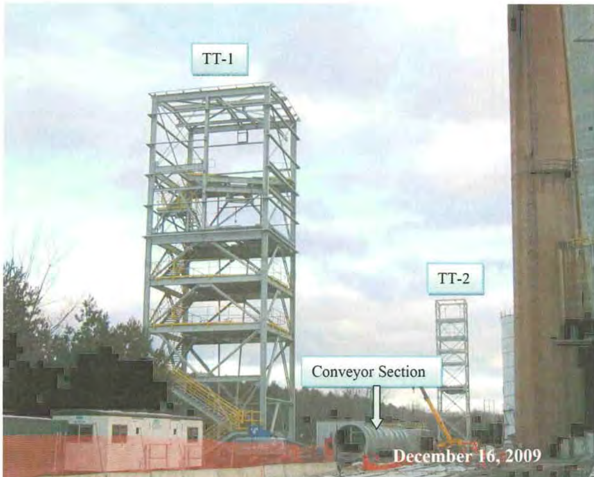
Figure 5. Limestone Transfer Tower 1 (foreground) and 2 (background)
