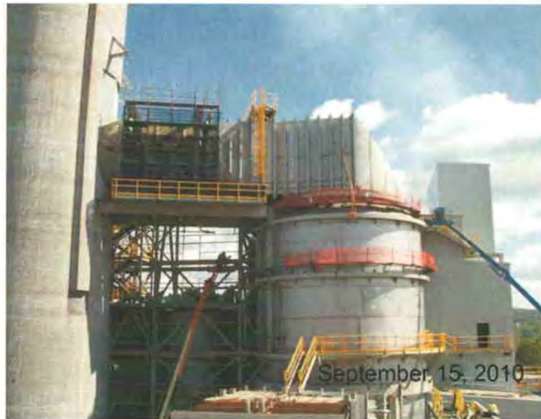
Figure 7 - Absorber Erection Progress – Installation of Outlet Hood and Transition Duct
