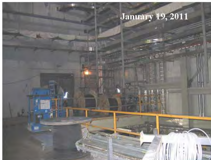
Figure A-6 Cable Pulling FGD Building
