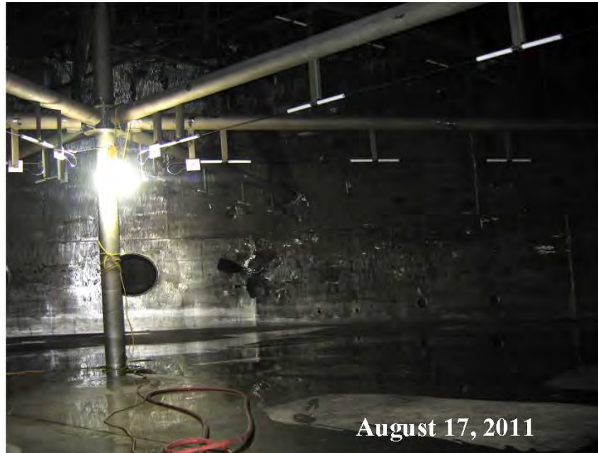
Figure A-5 PAP System Inside the Absorber
