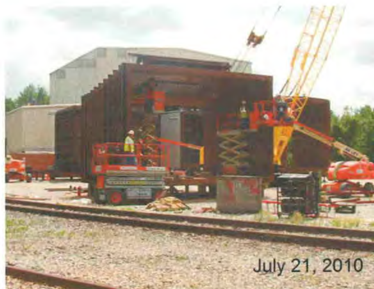
Figure A-8 - Flue Gas Ductwork Fabrication Area
