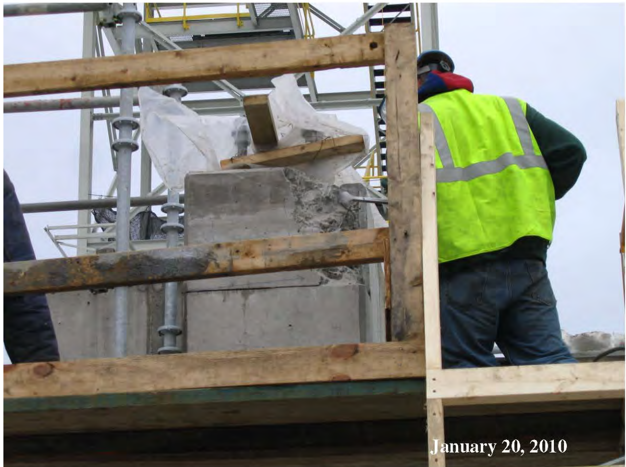
Figure 3 Repairing Limestone Ball Mill Foundation
