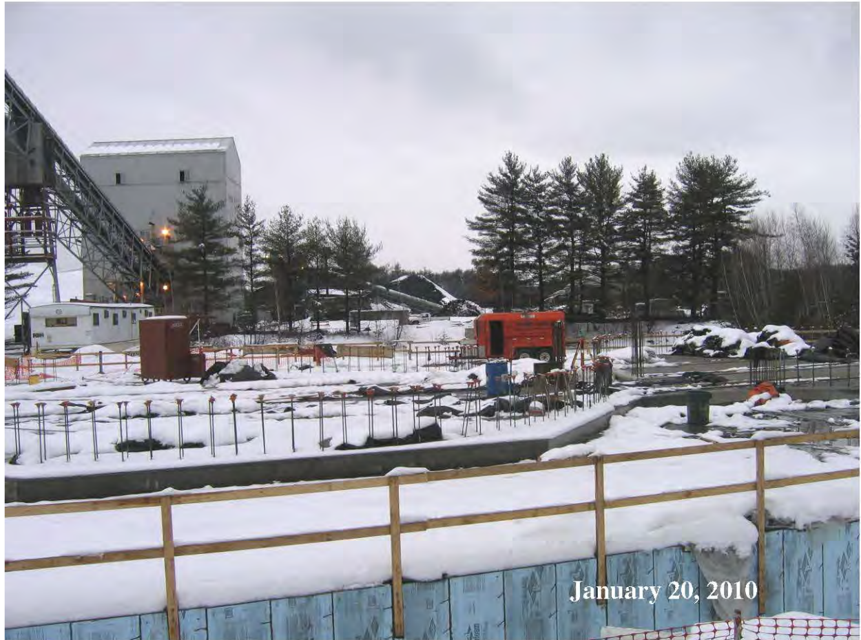
Figure 7 Limestone Silos Foundation After Concrete Placement
