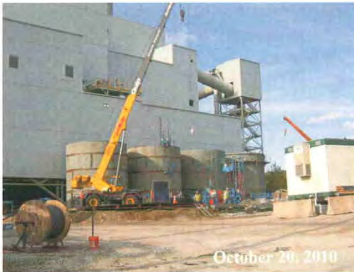
Figure A-4 South Side of FGD Building - Field Erected Tanks
