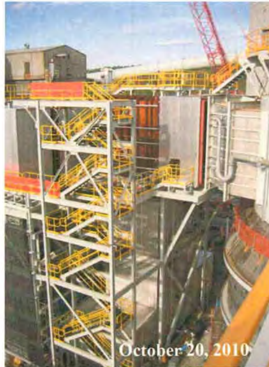
Figure A-2 BF Enclosure and FGD Inlet Duct
