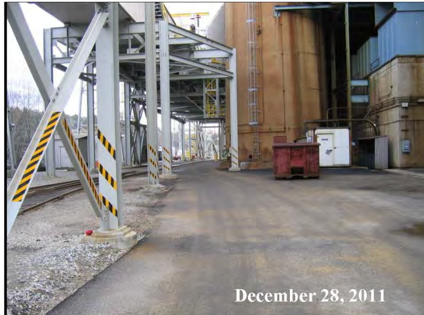
Figure A-7 Base Asphalt Paving
