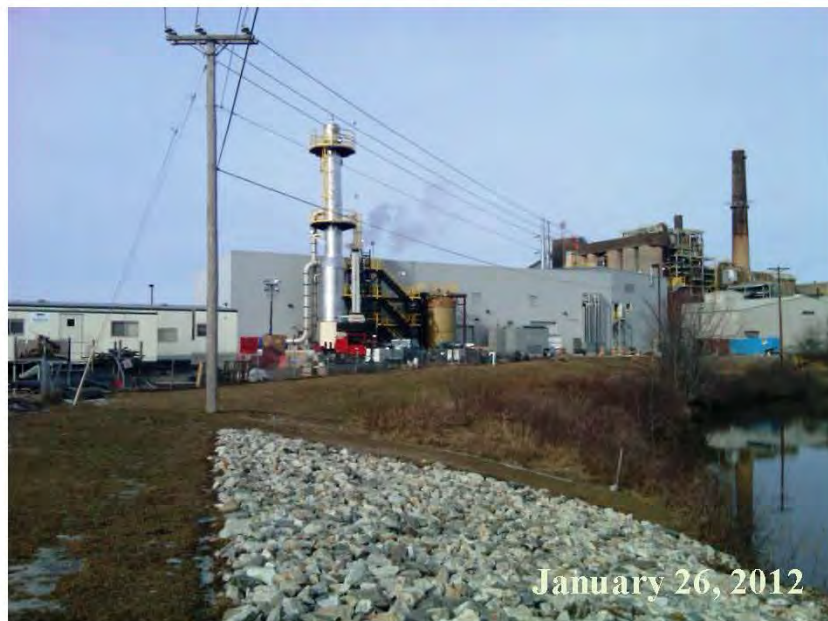
Figure A-2 SWWT Building Falling Film Evaporator
