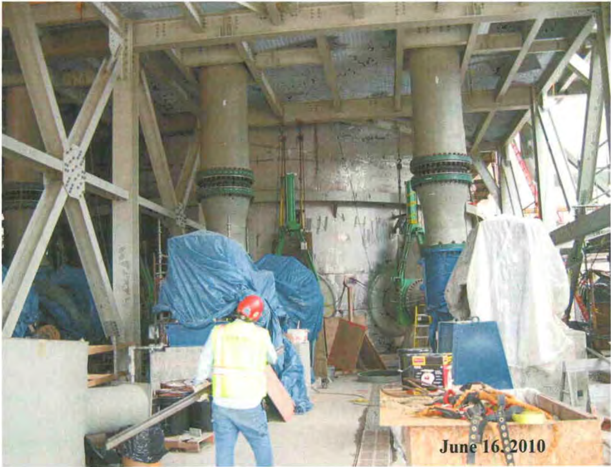
Figure 7 – Recycle Pumps and Piping
