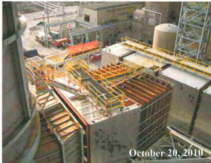
Figure A-5 Combined Flue Gas FGD Absorber Inlet Duct
