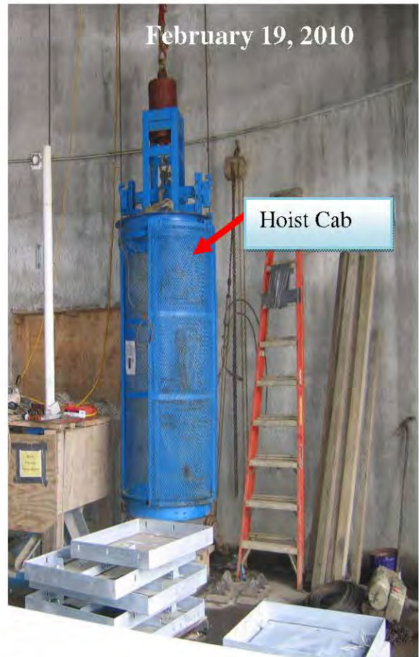
Figure 3 Chimney Hoist Drives and Cab (must be removed to install Booster Fan Foundation)
