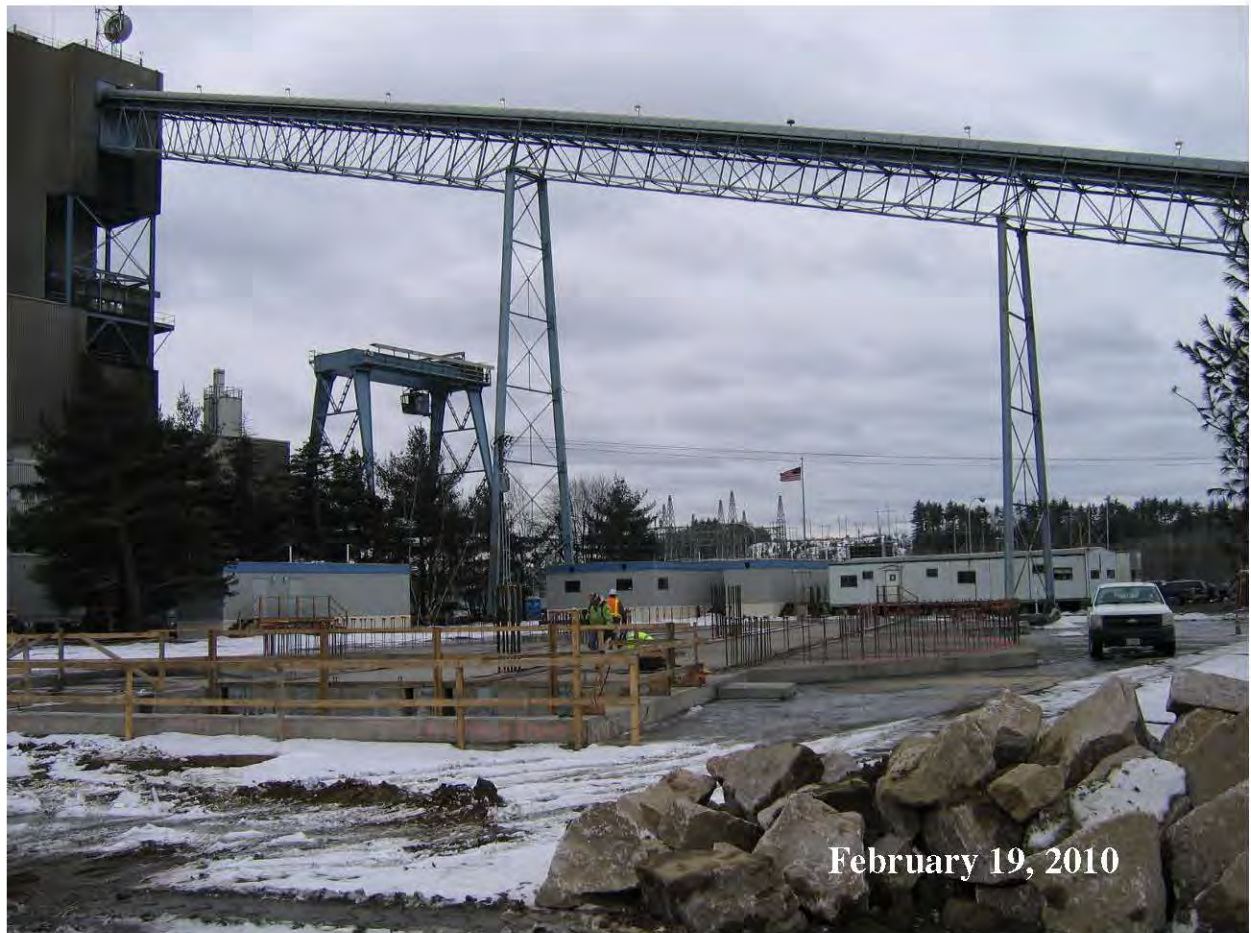
Figure 8 Limestone Silos Foundation
