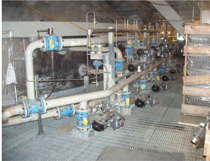
Figure A-5 Demister spray piping and valves
