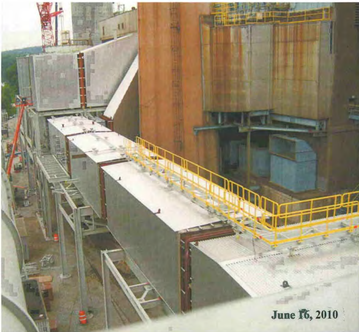
Figure 8 – Units 1 and 2 Flue Gas Ductwork
