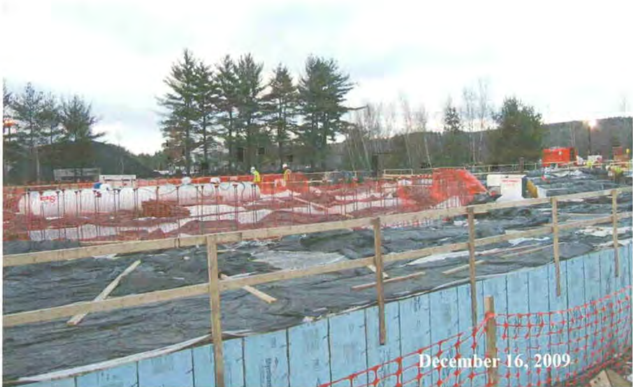
Figure 6. Limestone Silos Foundation Getting Ready for Concrete Placement
