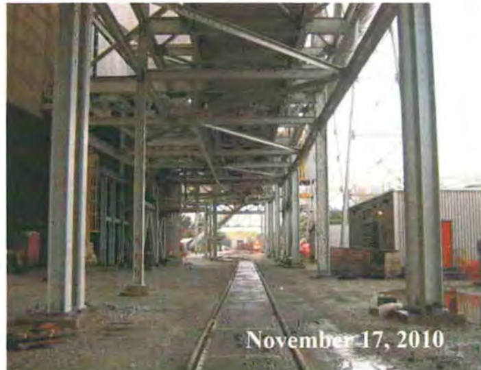
Figure A-5 Flue Gas Duct Support Steel and Unit 1 Duct Above
