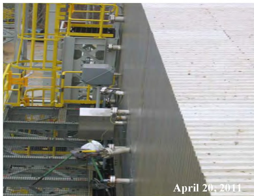
Figure A-8 Flue Gas Duct Penetrations and Instrumentation
