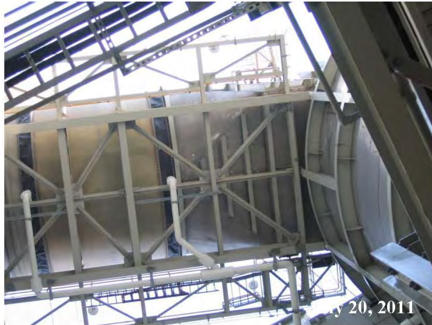
Figure A-7 Absorber Outlet Duct, Expansion Joints and Drain Piping
