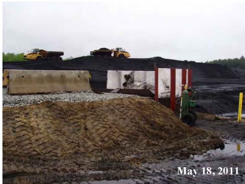
Figure A-6 Temporary Limestone Truck Unloading Ramp and Hopper in the Coal Yard
