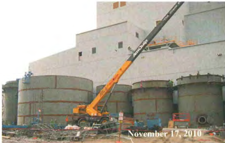
Figure A-7 FGD Building - South Side- Field Erected Tanks
