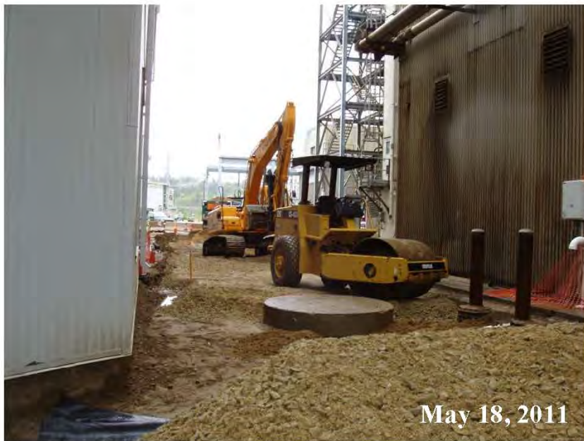
Figure A-4 GCC Installing Road Base for Paving between Booster Fan Enclosure and Existing Plant
