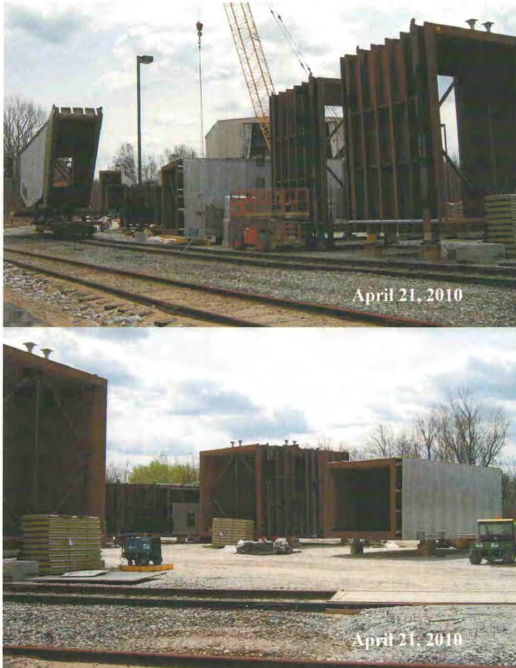
Figure 5 – Steel Duct Work Ground Fabrication
