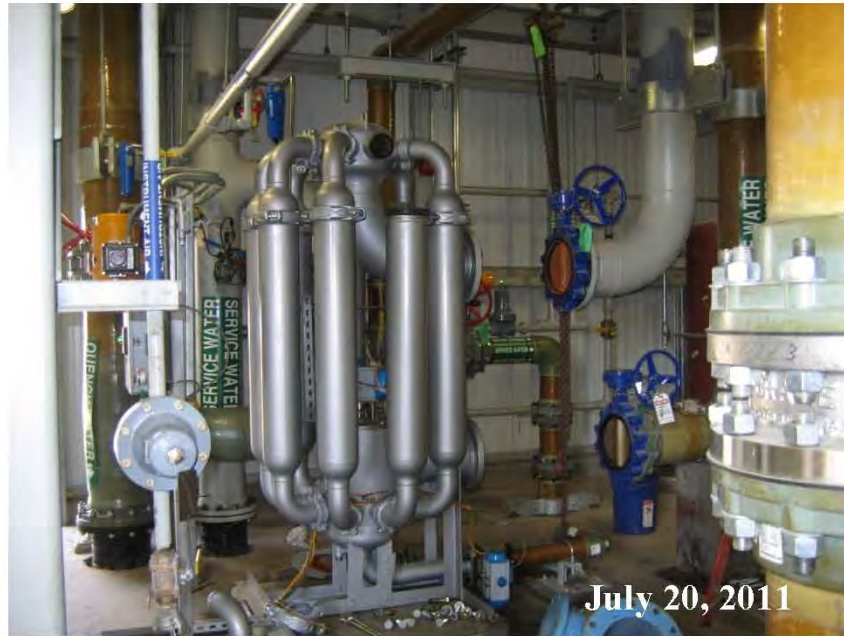
Figure A-11 Problematic (blinded) Service Water System Backwash Filter
