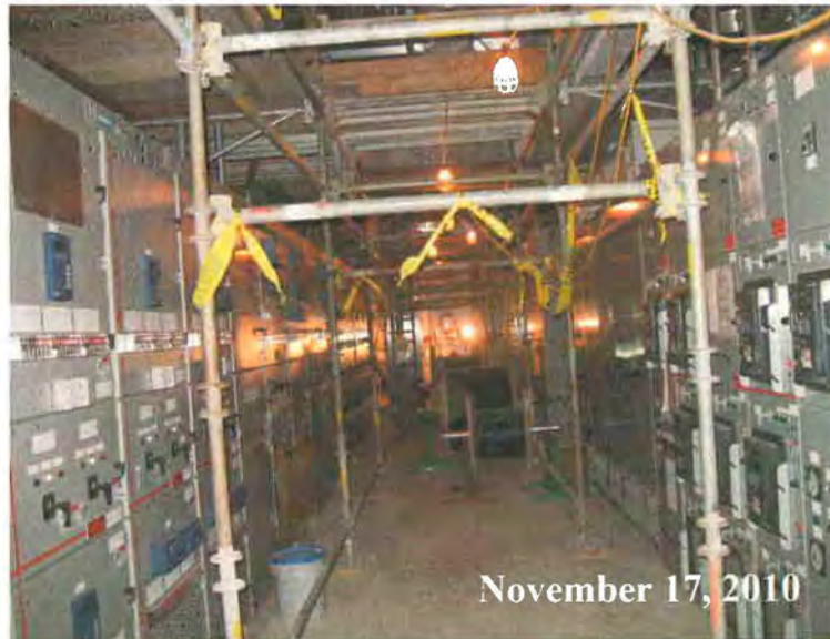
FigureA-10 FGD Electrical Room - Cable Pulling
