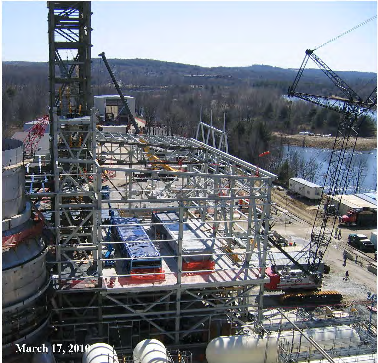
Figure 3 - FGD Building with Belt Filters Installed
