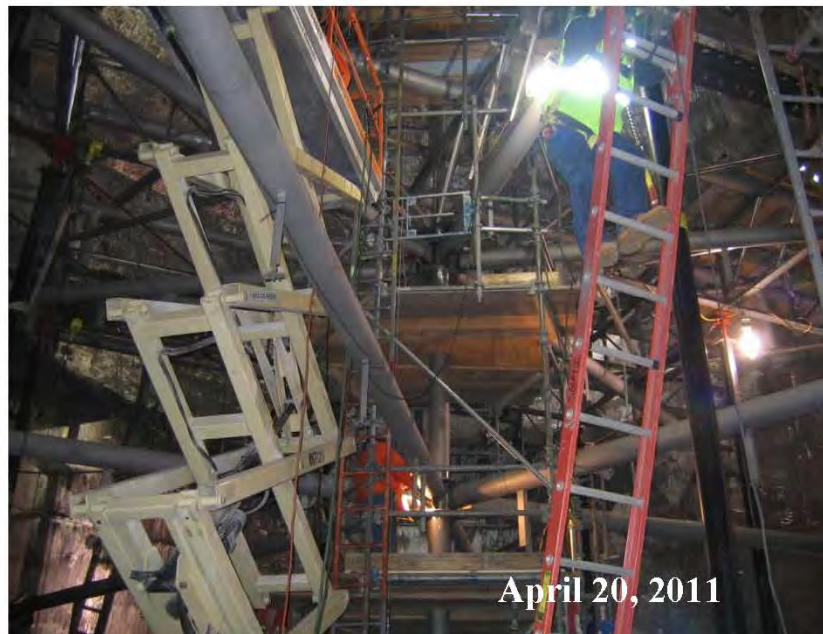
Figure A-6 Installation of the PAP System in the Absorber
