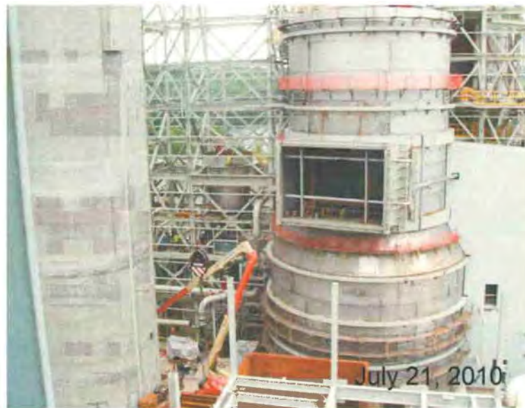
Figure A-7 - Absorber Erection Progress - Inlet
