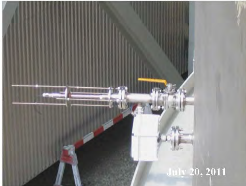
Figure A-5 PAP System Electrical Connection (near) – Analyzer Hot Tap Penetration (beyond)
