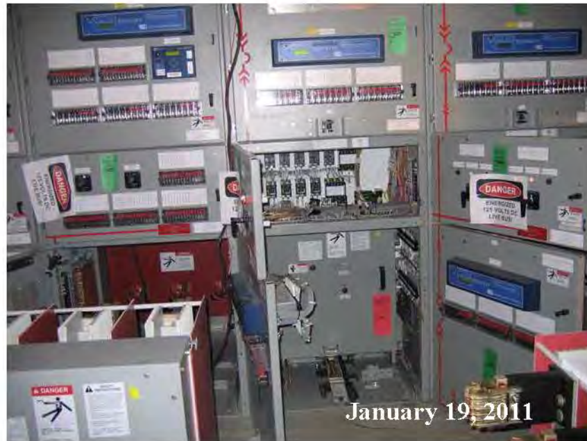
Figure A-7 Switchgear Terminations FGD Building Electrical Room
