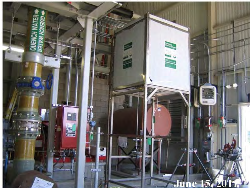
Figure A-12 L to R: Emergency Service Water Pump Diesel Drive, Diesel Storage Tank and Eye Wash
