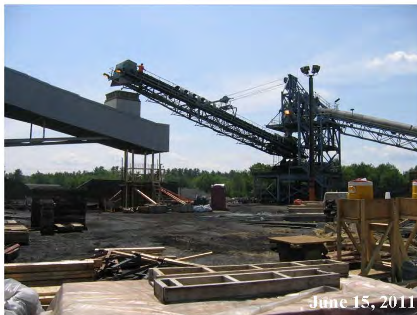
Figure A-10 Existing Radial Stacker and Limestone Receiving Hopper and Transfer Tower
