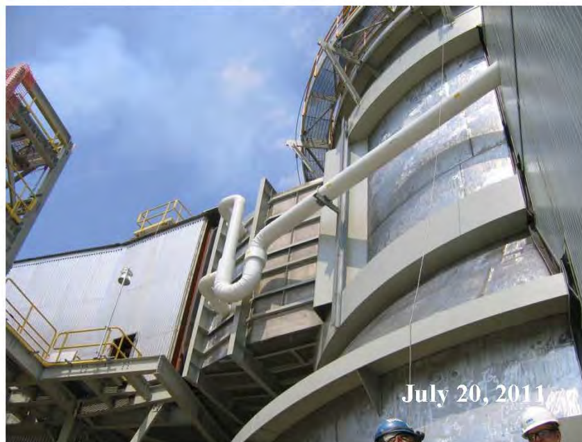
Figure A-6 Absorber Outlet Duct and Emergency Spray Piping
