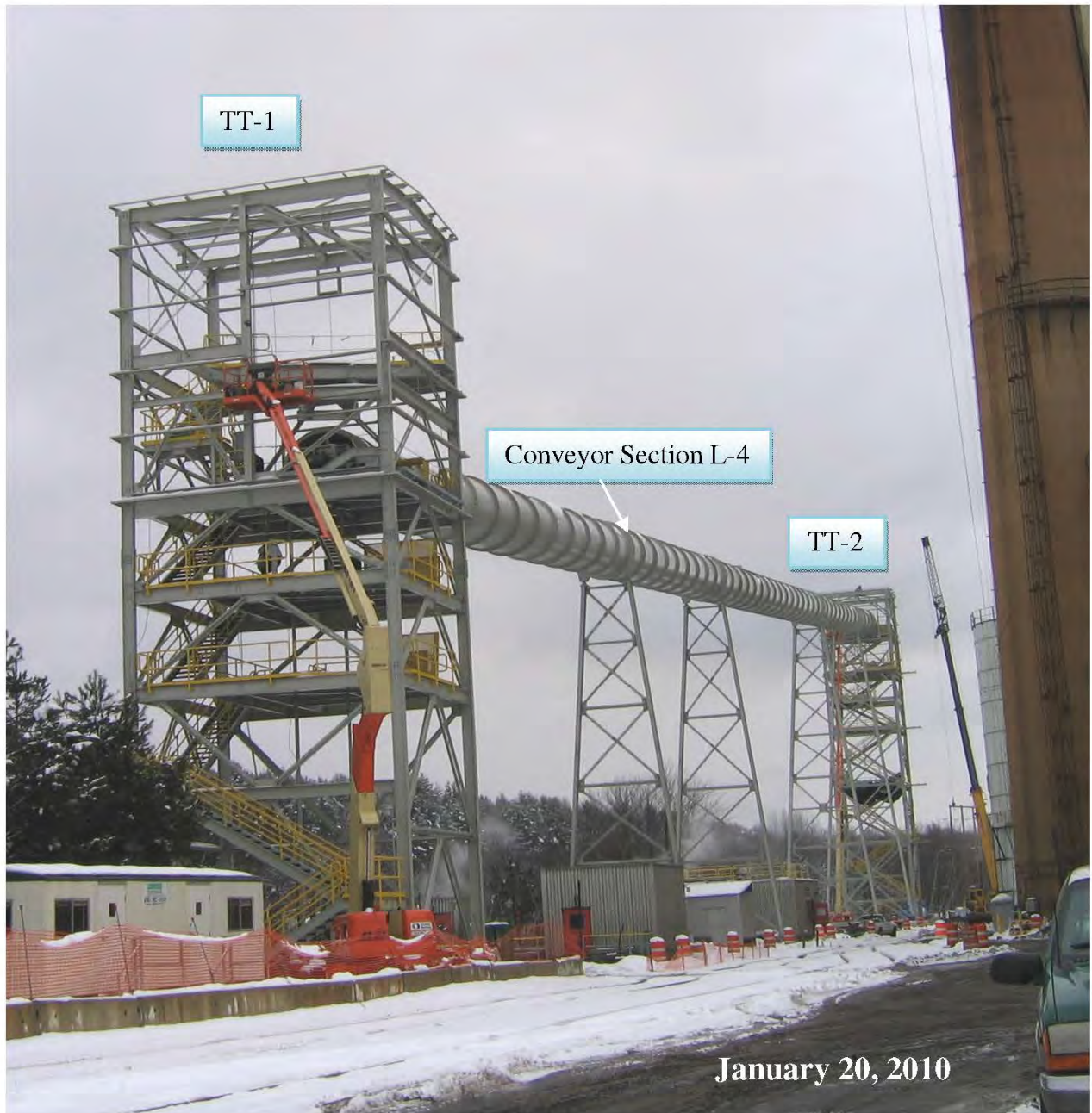
Figure 6 Limestone Conveyor L-4 and Transfer Towers 1 (left) and 2 (right)
