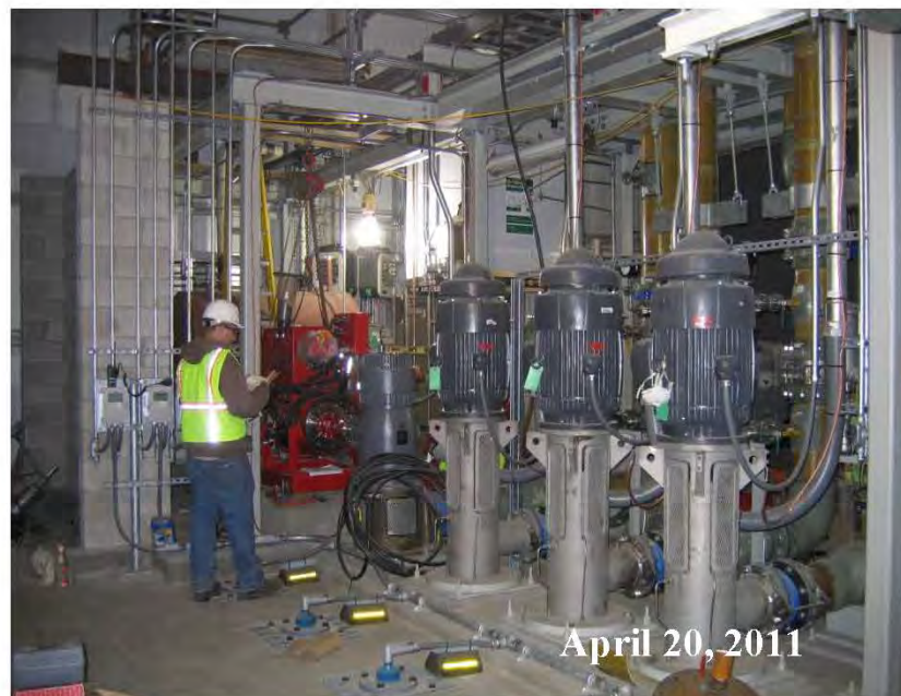
Figure A-2 Service Water Pumps and Red Emergency Diesel Quench Pump
