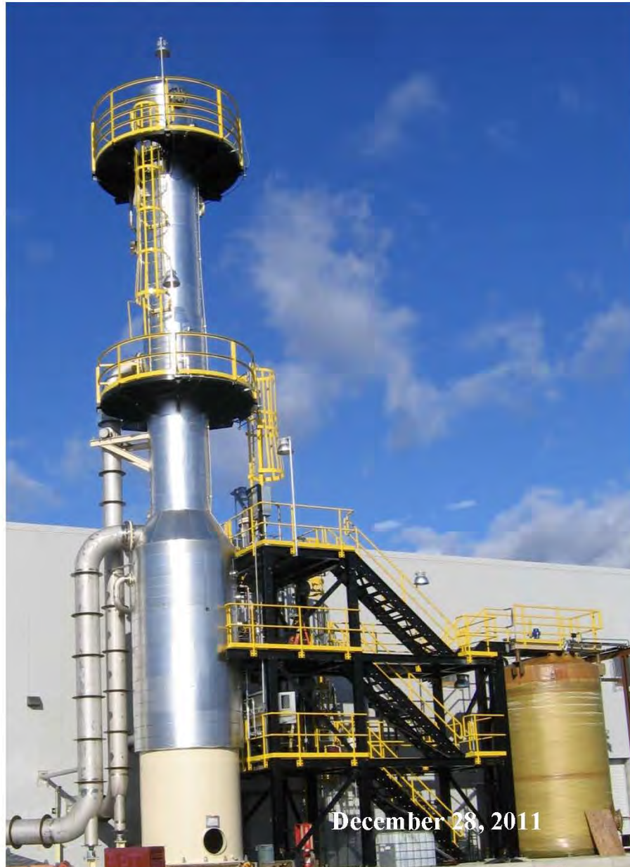
Figure A-2 SWWT System Falling Film Evaporator
