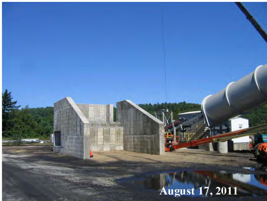
Figure A-8 Limestone Truck Unloading System
