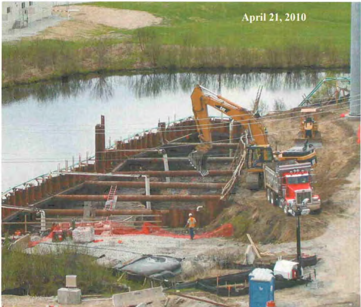
Figure 6 – Excavation for the Service Water Pump House Foundations
