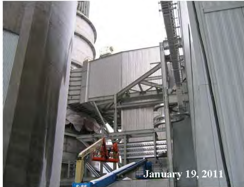
Figure A-3 Outlet of Booster Fans and Inlet of FGD Absorber
