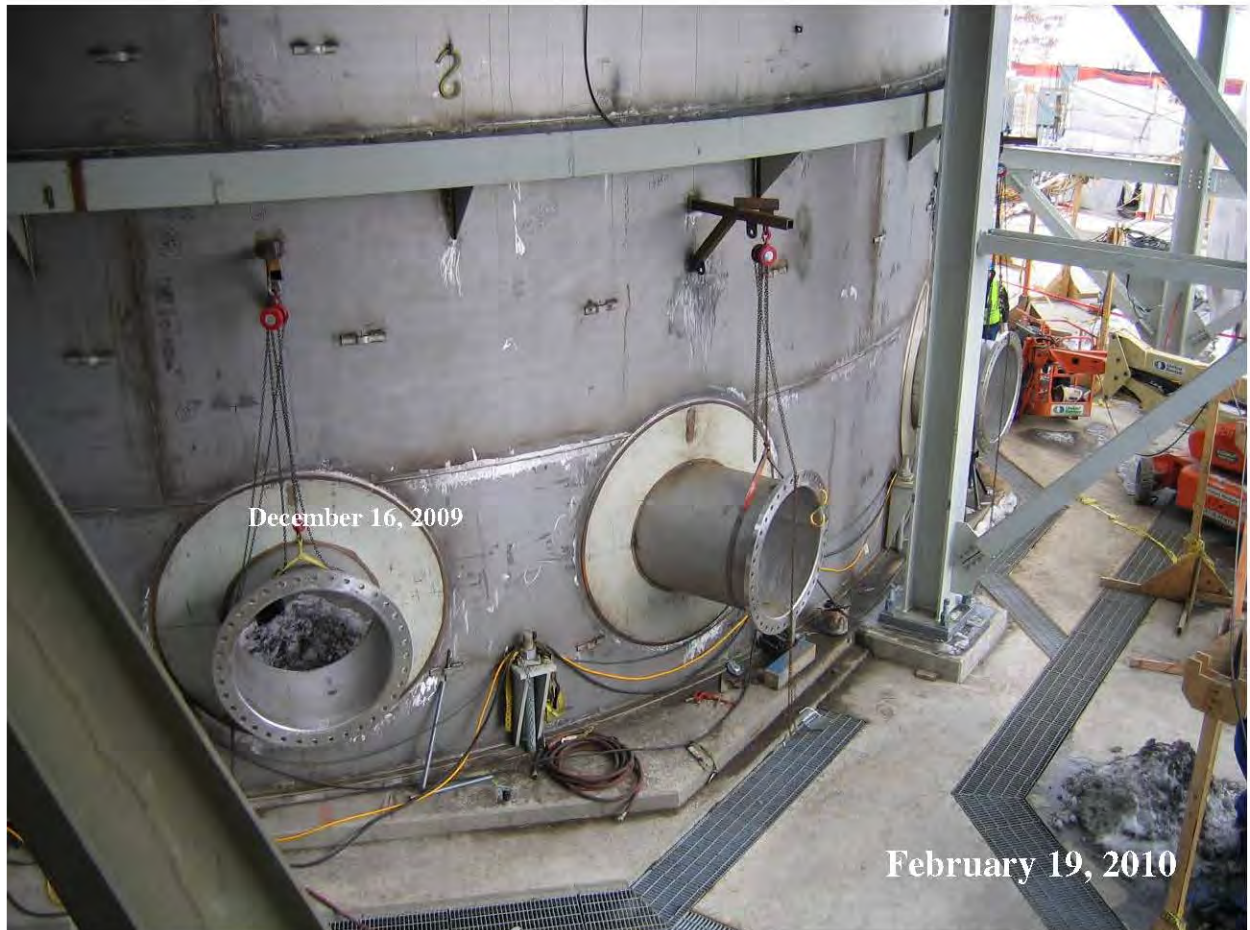
Figure 6 Absorber and Recycle Nozzles
