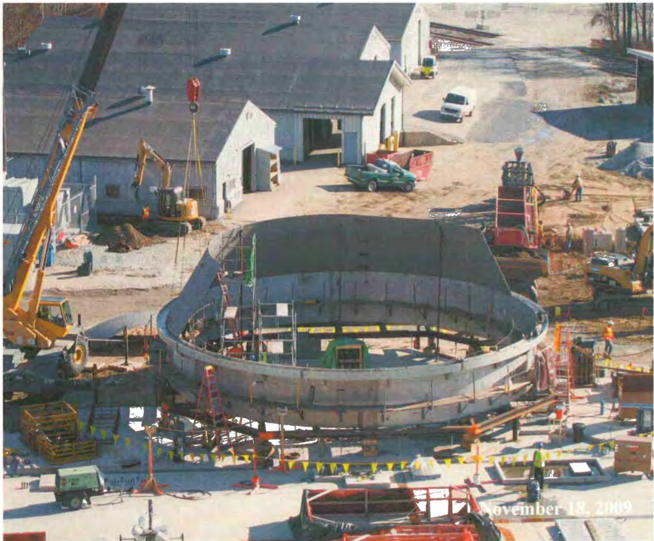
Figure 3. Absorber Fabrication Table
