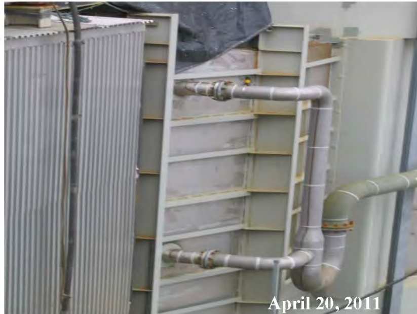
Figure A-7 Absorber Inlet Duct, Expansion Joint and Emergency Spray Piping
