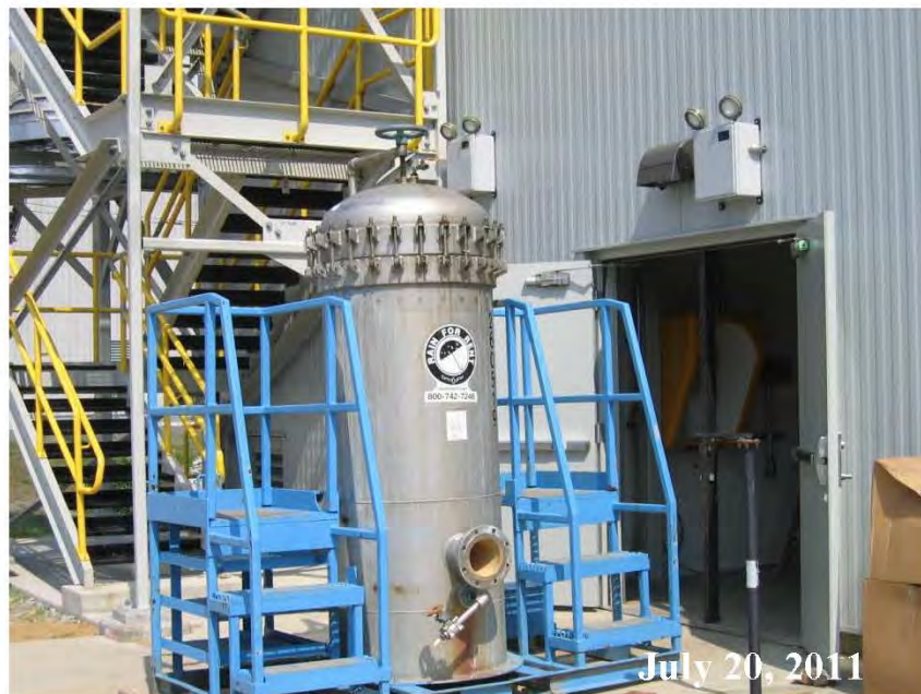
Figure A-12 Temporary Replacement for the Backwash Filter
