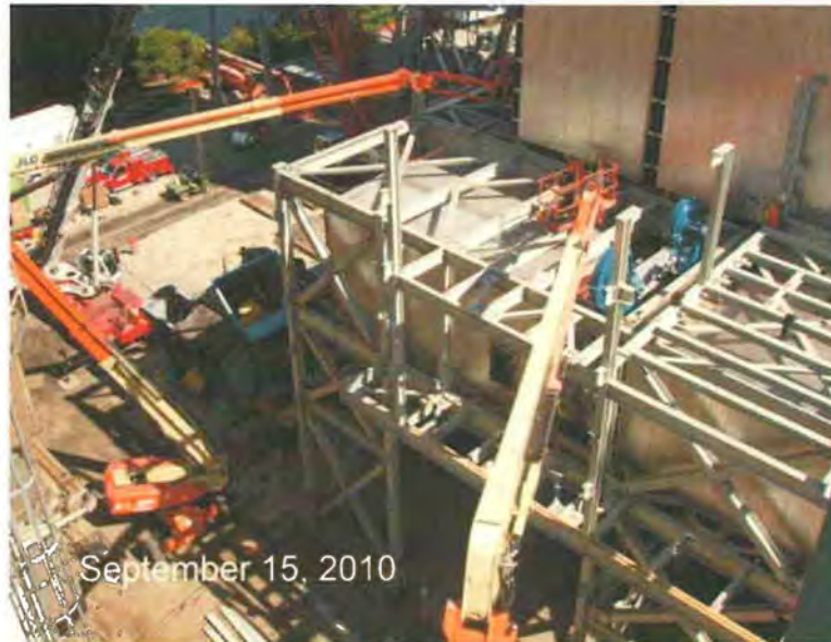
Figure 5 - Unit 2 BF Casings (left) Unit 2A Duct Support Steel (right)
