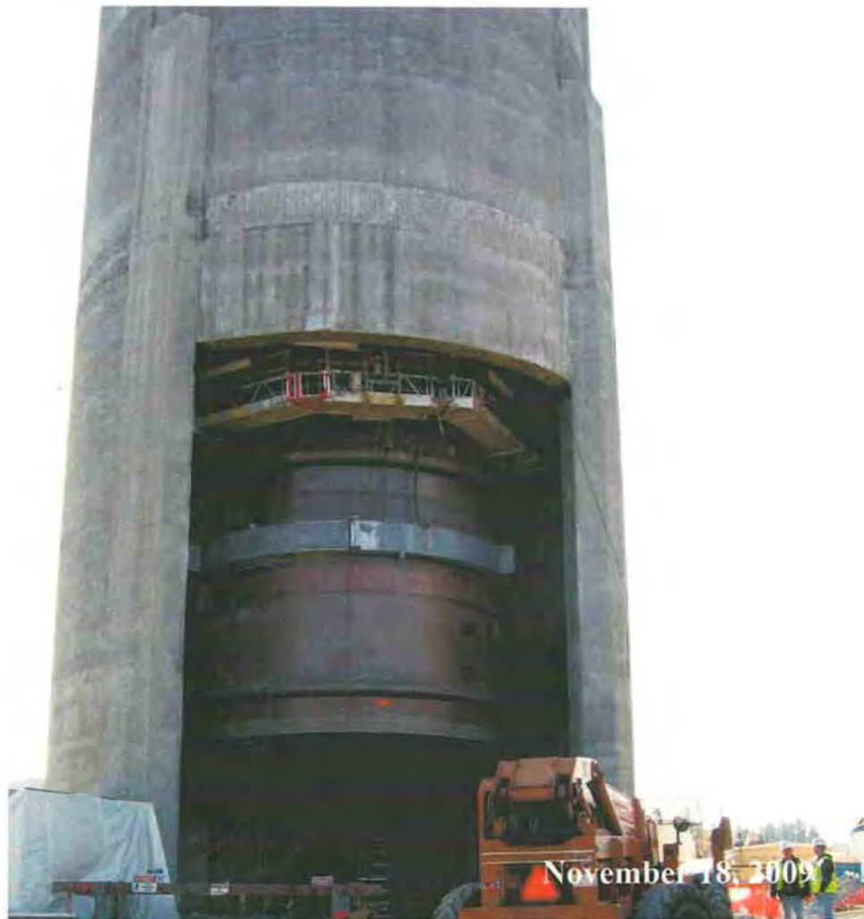
Figure 5. Chimney Showing Liner Can Installation
