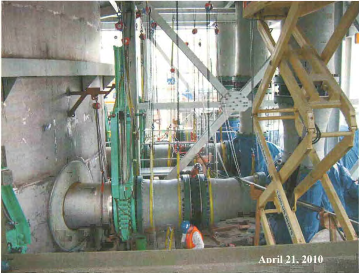
Figure 8 – Absorber Recycle Fiberglass Piping
