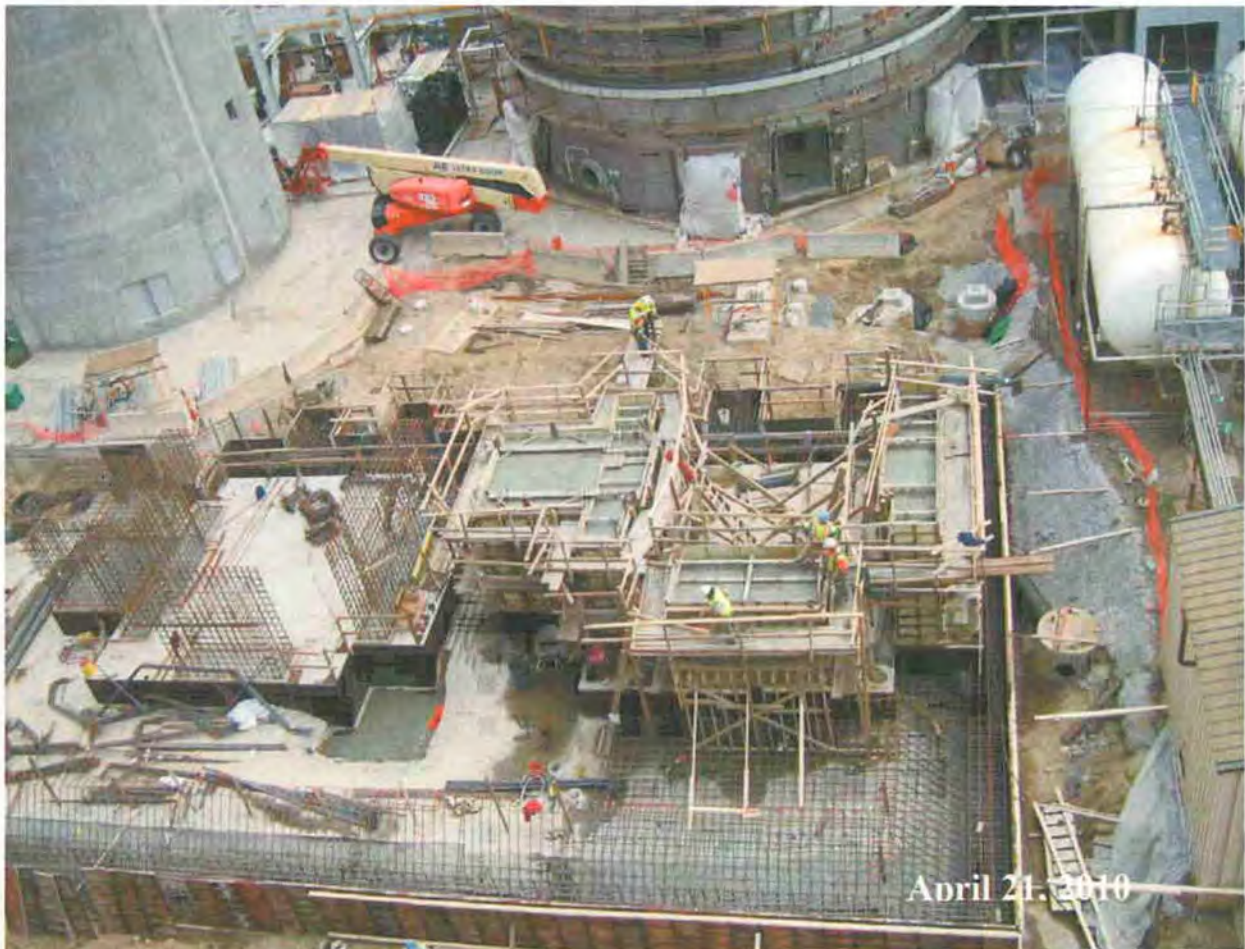
Figure 7 – Foundations for the Booster Fans and Enclosure
