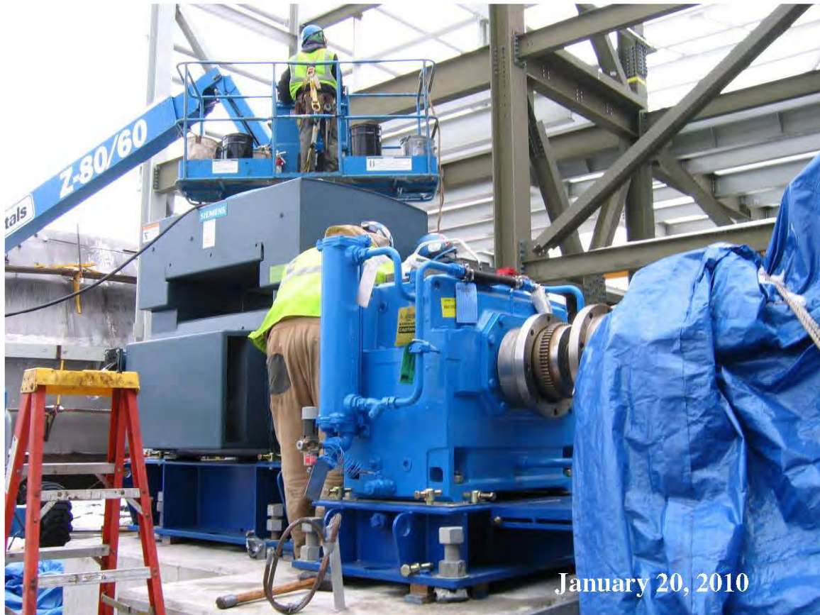
Figure 2 Recycle Pumps
