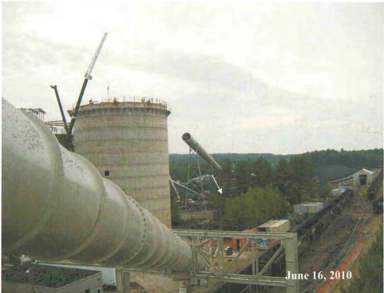
Figure 9 – Limestone Conveyors L-2 and L-3
