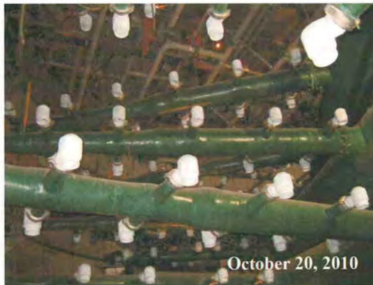
Figure A-8 Absorber Spray Nozzles and Headers
