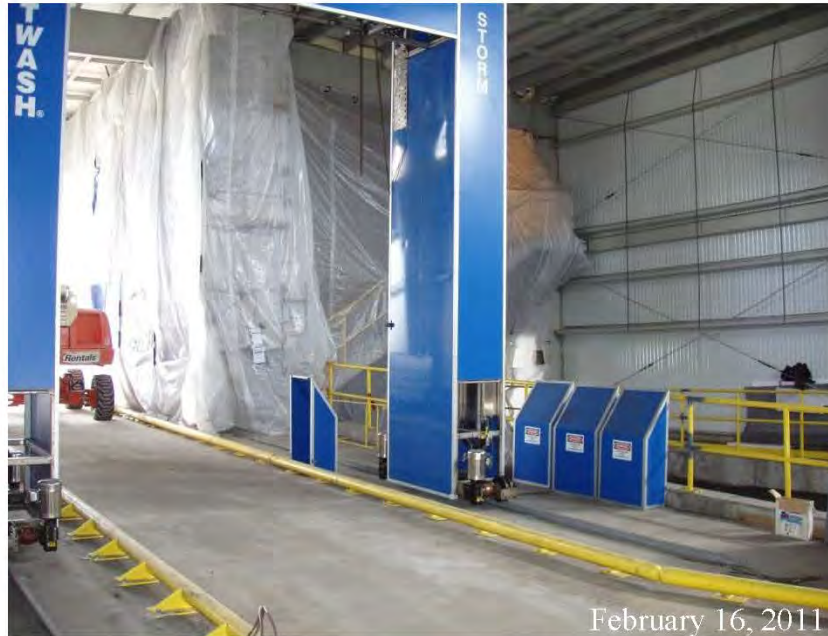
Figure A-9 Inside Truck Wash – Installation of Mechanical Equipment and Block Walls
