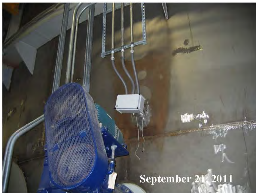
Figure A-4 Electrical Connections to PAP System Absorber Penetration
