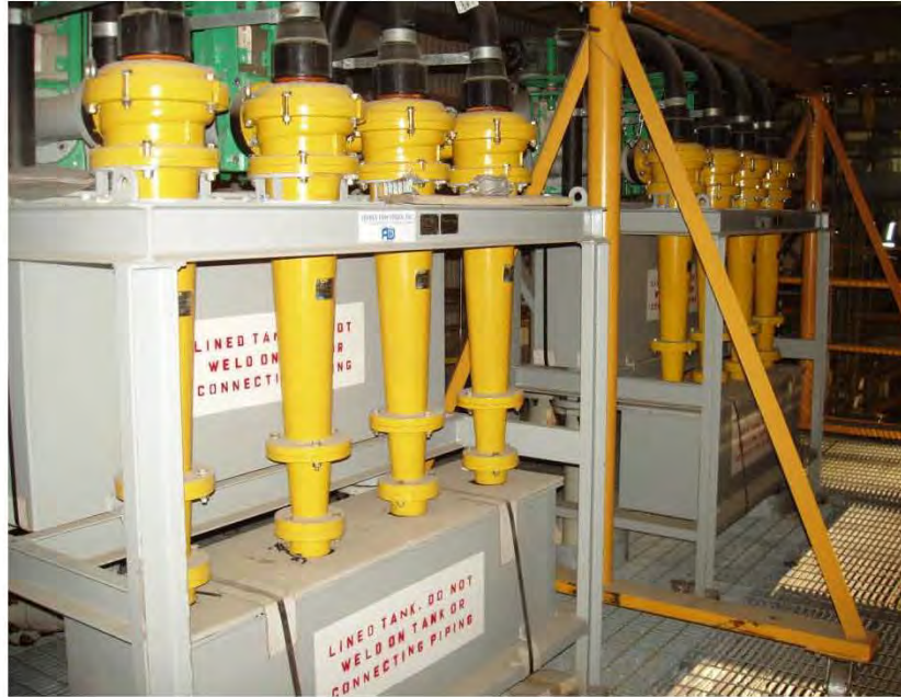
Figure A-7 Hydroclones inside FGD Building
