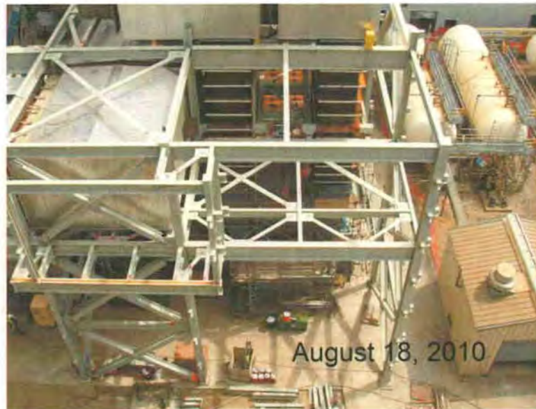
Figure A-6 - Booster Fan and Enclosure - West End
