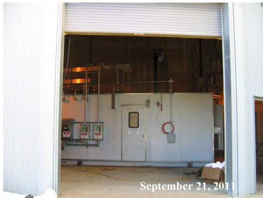
Figure A-6 CEMS Trailer at the Base of the Concrete Chimney
