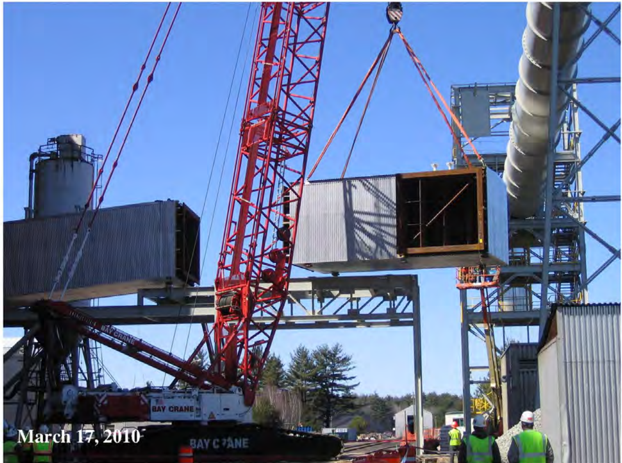
Figure 6 - Installation of Unit 1 Flue Gas Steel Ductwork
