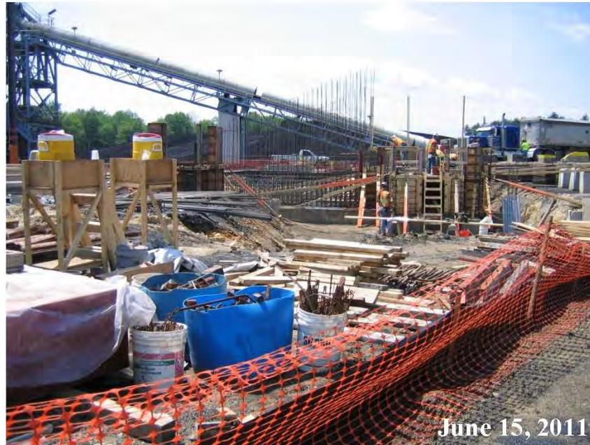
Figure A-9 Limestone Truck Unloading Foundations
