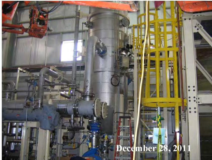
Figure A-3 SWWT System Crystallizer
