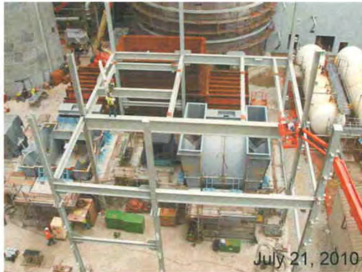
Figure A-5 - Unit 2 Booster Fan Foundations, Casings and Ductwork
