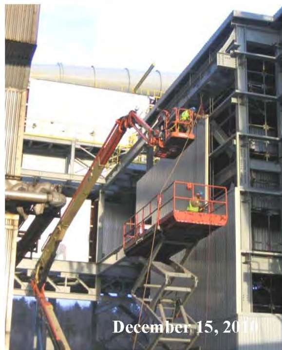
Figure A-8 FGD Booster Fan Enclosure Siding
