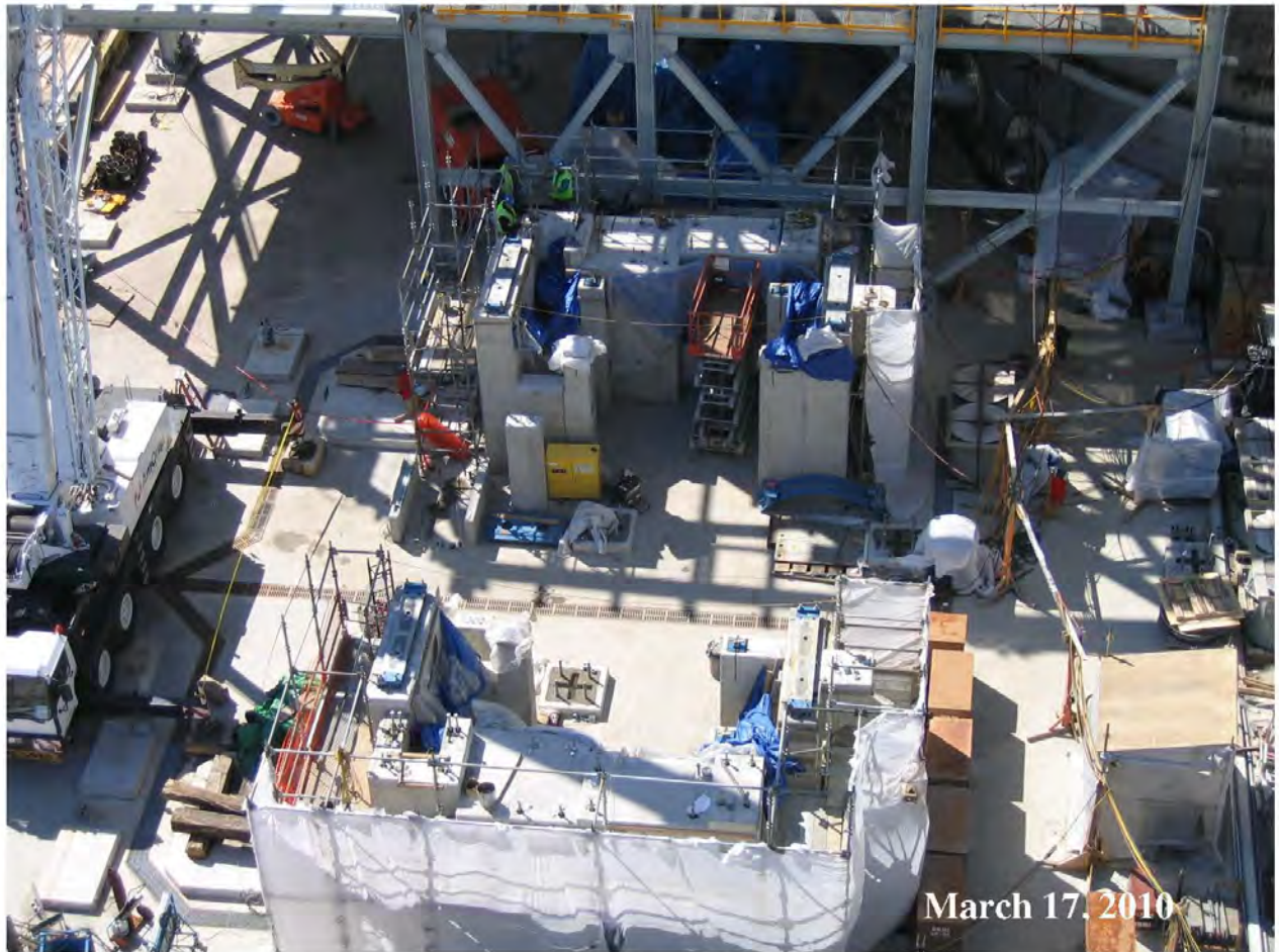
Figure 7 - Ball Mill Foundations
