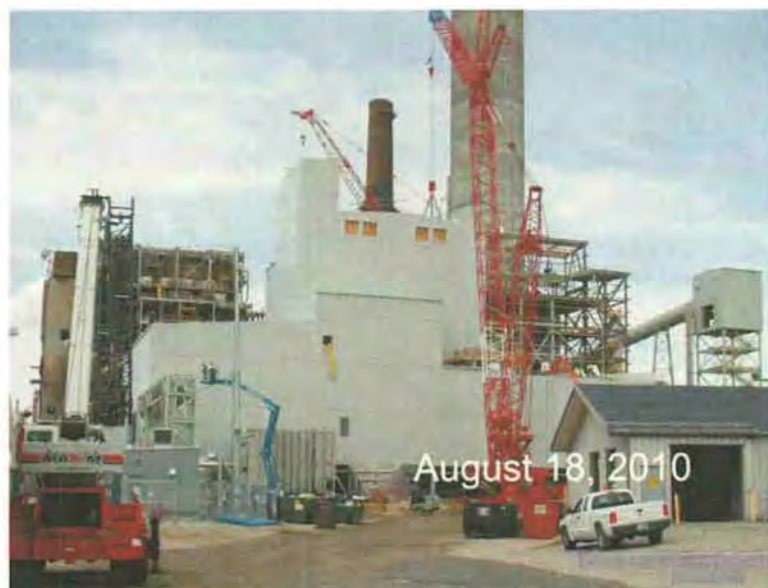
Figure A-3 - Gypsum Building - Stackout Conveyors
