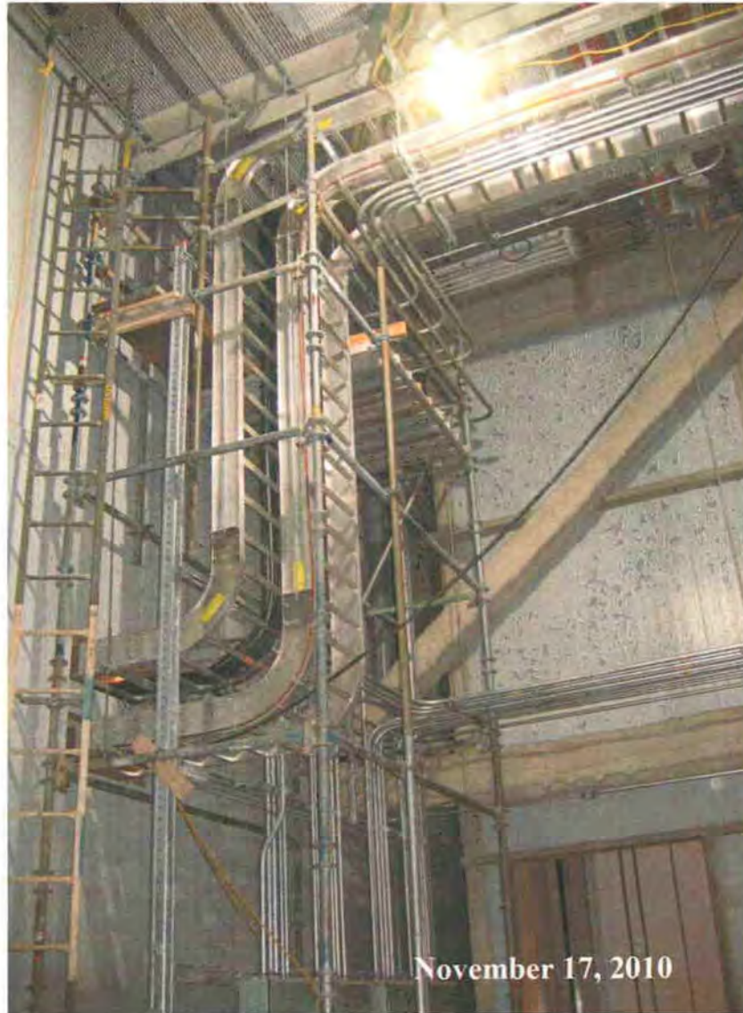
Figure A-9 Cable Tray and Conduit - FGD Building
